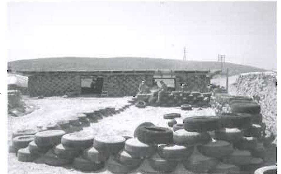
Al Khan Al Ahmar primary school, Palestine, building with tyres / Al Khan Al Ahmar basisschool, Palestina, bouwen met autobanden
