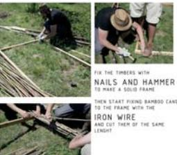
FIX THE TIMBERS WITH NAILS AND HAMMER TO MAKE A SOLID FRAME
