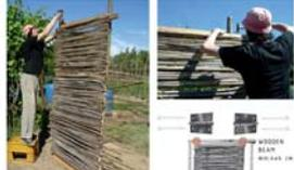
USE NAILS, HAMMER AND PIVOTS TO FIX YOUR SHADING PANEL TO THE EXTERNAL WOODEN BEAM OF YOUR WALL
